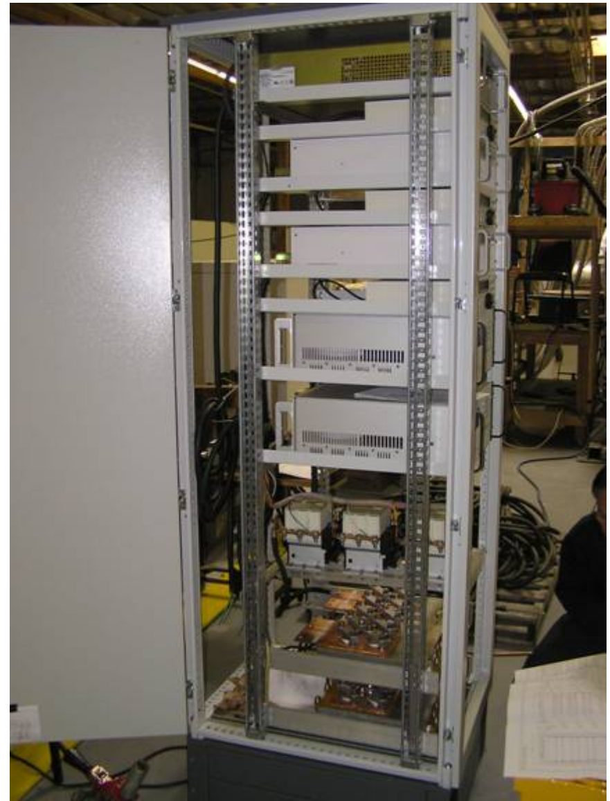
Front and rear views of assembled RAL racks for powering a single Spectrometer Solenoid
