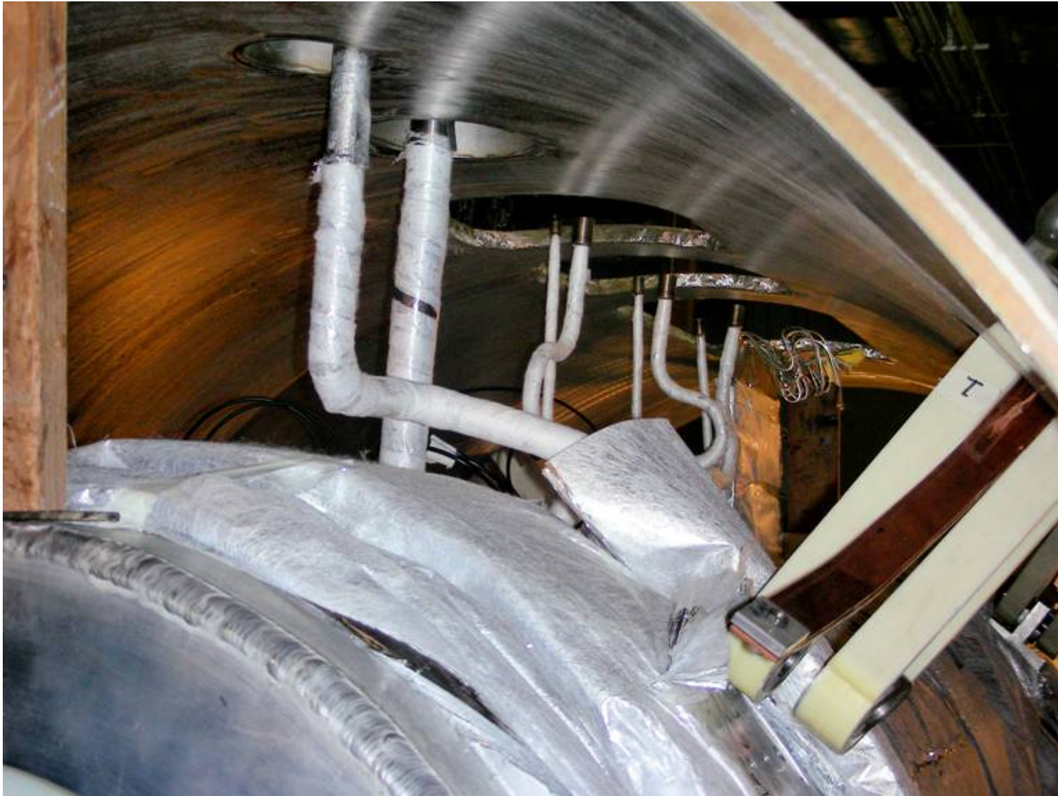
Cold mass connections during assembly into vacuum vessel (Magnet 1, 1 st iteration)
