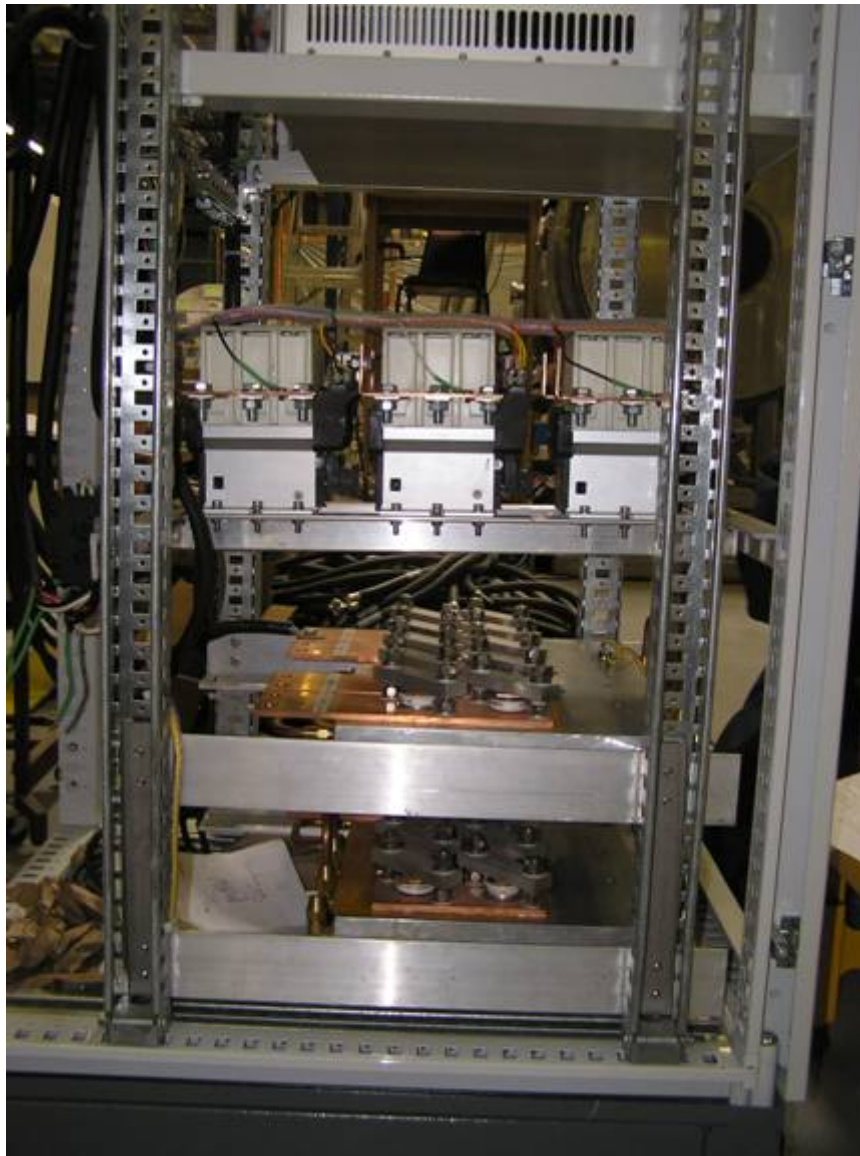
Front and side views of switches and power absorbing blocks for magnet discharge circuits
