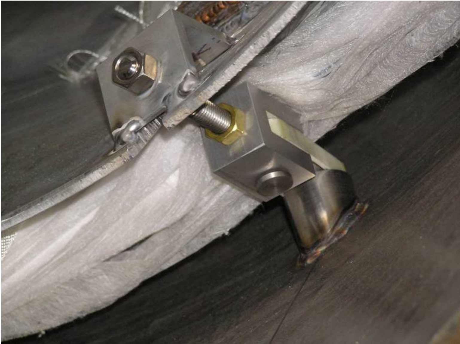
Overall view of installed thermal shield support
