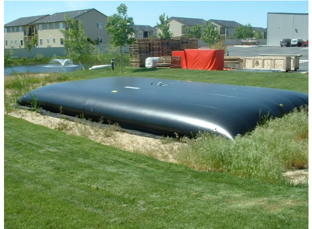
Figure 7.13: Flexible fuel bladder like this one can be used as a last level of security in the highly unlikely event that all the other safety measures to prevent the loss of enriched ^{136}\text{Xe} to the atmosphere fail.
