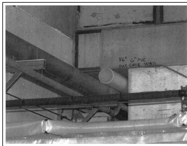
Figure 32. Vent piping exit outside the cave. The 6-inch PVC pipe is 86-inches long through the cave wall to discharge.
