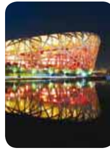
CHINA Beijing National Stadium
