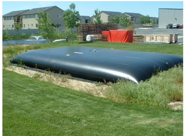
Figure 8.12: Flexible fuel bladder like this one can be used as a last level of security in the highly unlikely event that all the other safety measures to prevent the loss of enriched ^{136}\text{Xe} to the atmosphere fail.
