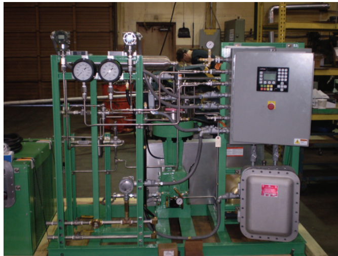
Figure 8.9: Example of the re-circulation pump chosen for the Xe purification gas system. This is a triple stainless steel diaphragm pump capable of 100 slpm flow rates.
