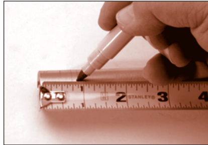
FIGURE 57: Measuring depth of insertion
