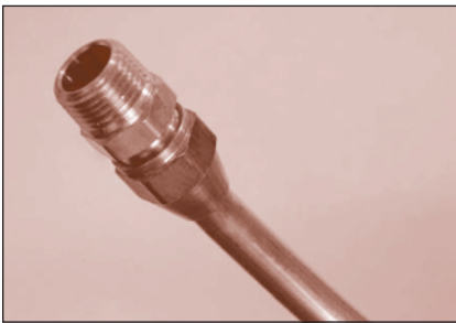
FIGURE 29: Completed flared joint
