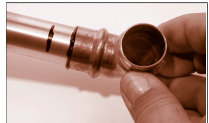
FIGURE 89: Visual check of adhesive coverage
