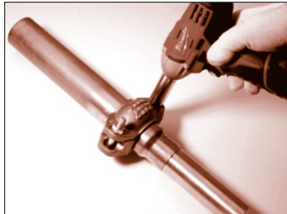
FIGURE 43: Tightening the clamp
