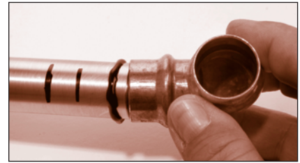
FIGURE 87: Inserting tube end
