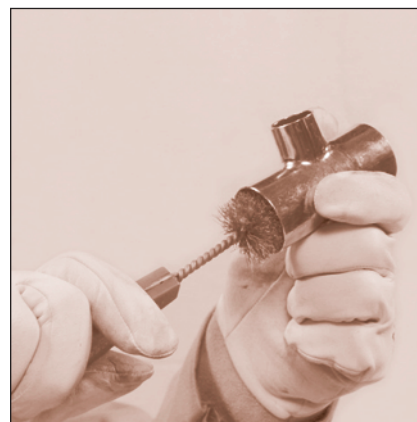
FIGURE 17: Cleaning: Fitting brush
