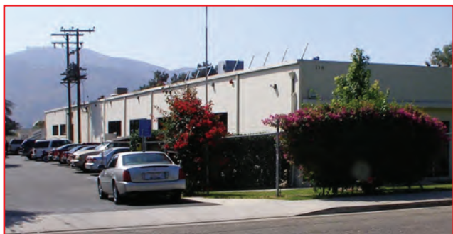
ARP's new forging facility in Santa Paula, California.
