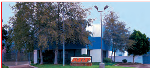
All metal finishing operations are done in this Santa Paula plant.
