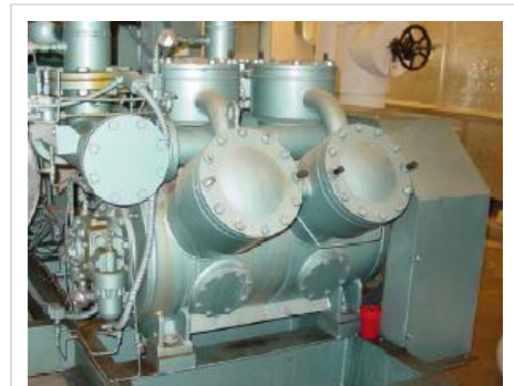
A motor-driven six-cylinder reciprocating compressor that can operate with two, four or six cylinders.
