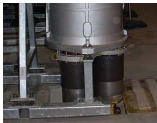
Fig. 5: example of 170 kV dry outer cone termination.
