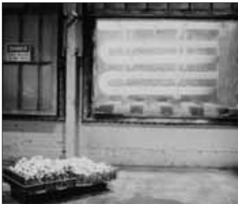
Figure 2.4. 253 MA radiant tubes in a heat treatment furnace. Courtesy of Rolled Alloys.
