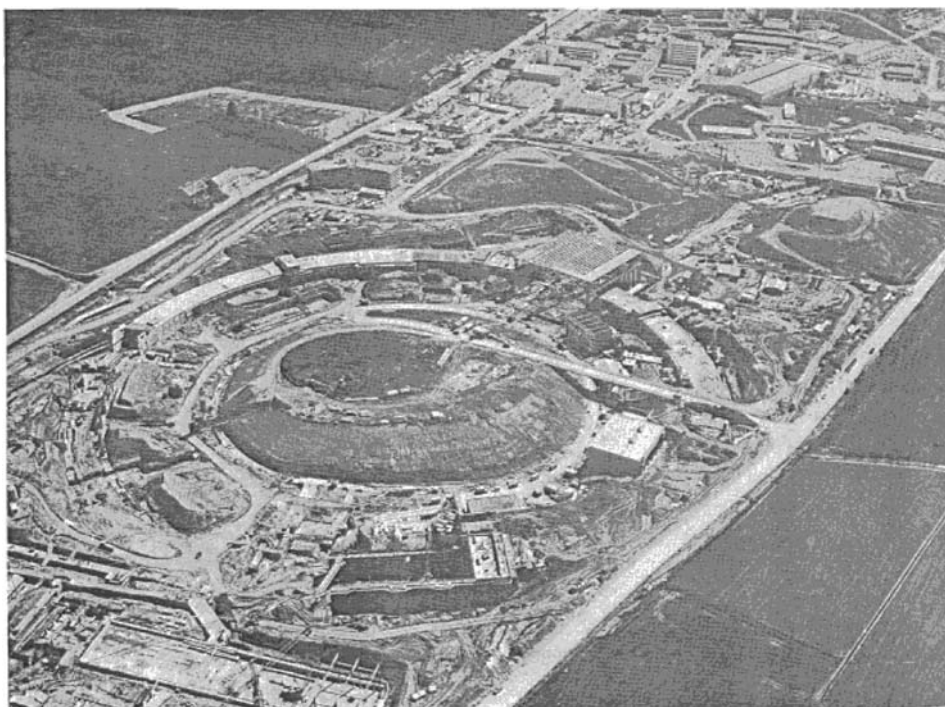
Fig. 7.25 State of construction in April 1969. In the foreground, work has started on the building housing the control room, and also on the Experimental Hall 14. To the right, Octant 3 is already being covered and the tunnel is complete as far as Octant 7. On the far side, the steel work for Hall 11 is in position and in the background the tunnel of the booster is about half complete. Top right is the PS itself. (Courtesy of CERN).
